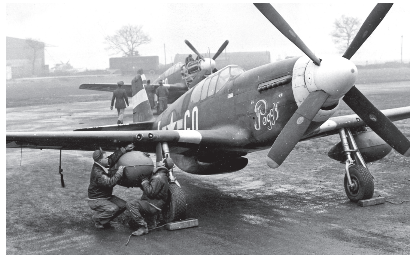
Below: C-51B Mustang s/n 43-12451 GQ+I Peggy has 75-gallon drop tanks fitted on by Sgt. Segar and SSgt. Smith at Boxted, England, during April 1944. “Peggy” was SSgt Smith’s wife while the left side of the P-51B carried the name Live Bait! (Photos courtesy of Jack Cook)
